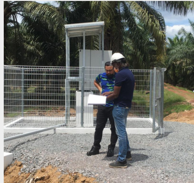
River NH3 Monitoring Station (2020 ~ 2022)
